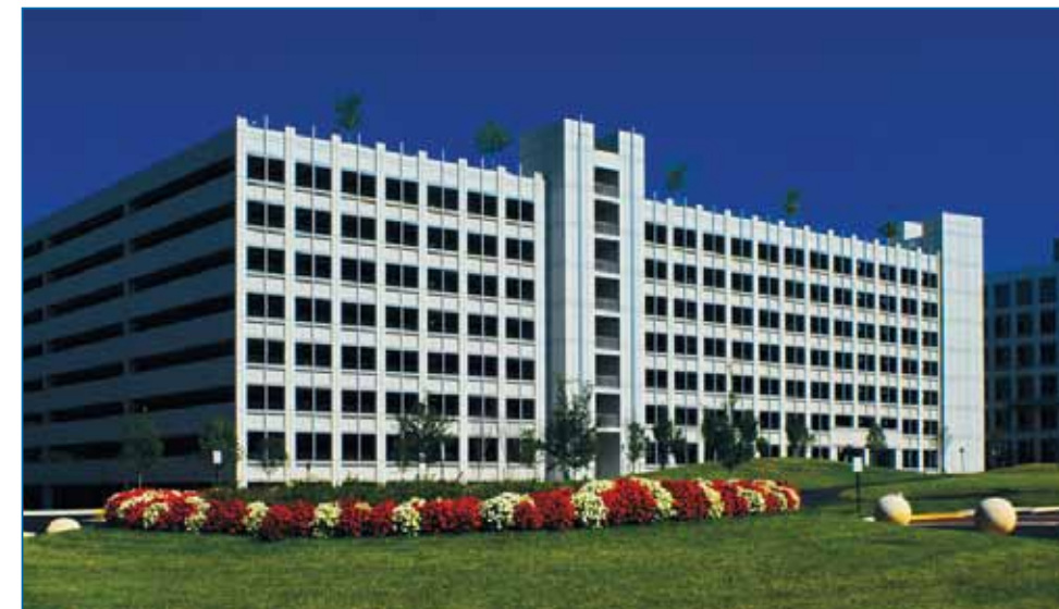
Dulles Station Parking Deck in Herndon, VA
