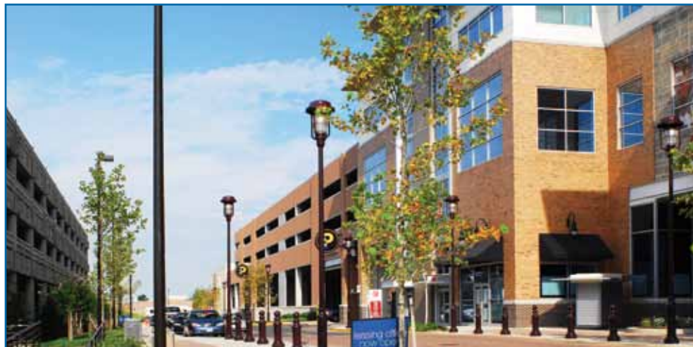
Belcrest Center Retail/Parking Structure in Hyattsville, MD
