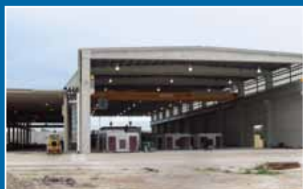
Six-sided, dual cell modules in production at Tindall's new San Antonio plant.
